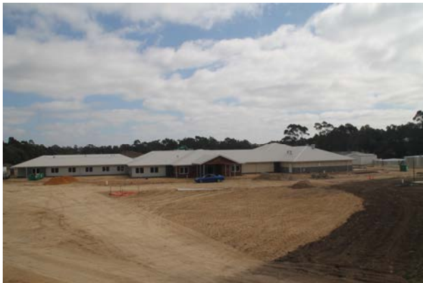
View to the front of the building at the end of 2019
